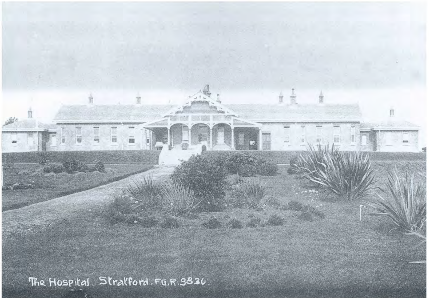
"The ex-hospital clay roof tiles dependably keep out the weather and add to the permanent appearance of the villas." - Helen Mays, Manawatu Evening Standard, Oct. 2001
